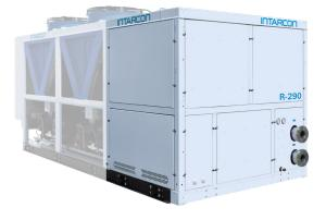
Pump sets for water or glycol in closed circuit, assembled in galvanised sheet steel bodywork and structure with polyester paint for outdoor installation and coupled to the chillers.
